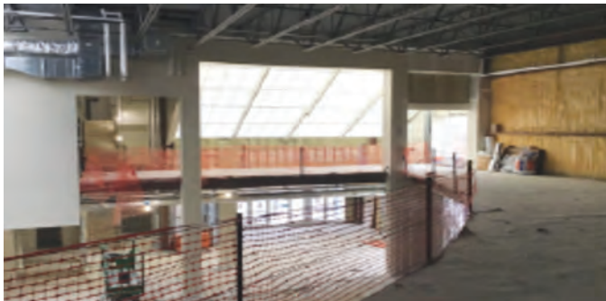
3. Second Floor View of the Lobby and Display Area
