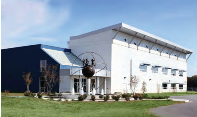
1. DASEF Innovation Technology Exploration Center (ITEC)
