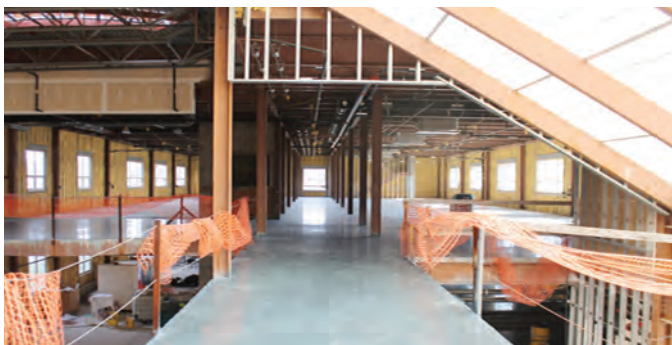
7. Polished Cement Walkways on all Hallways and Upper and Lower Display Areas
